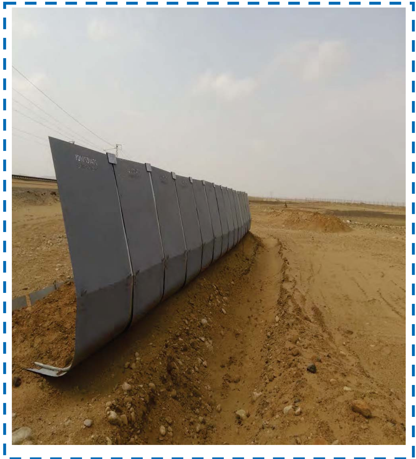
Desert Sand Trap at installation time
