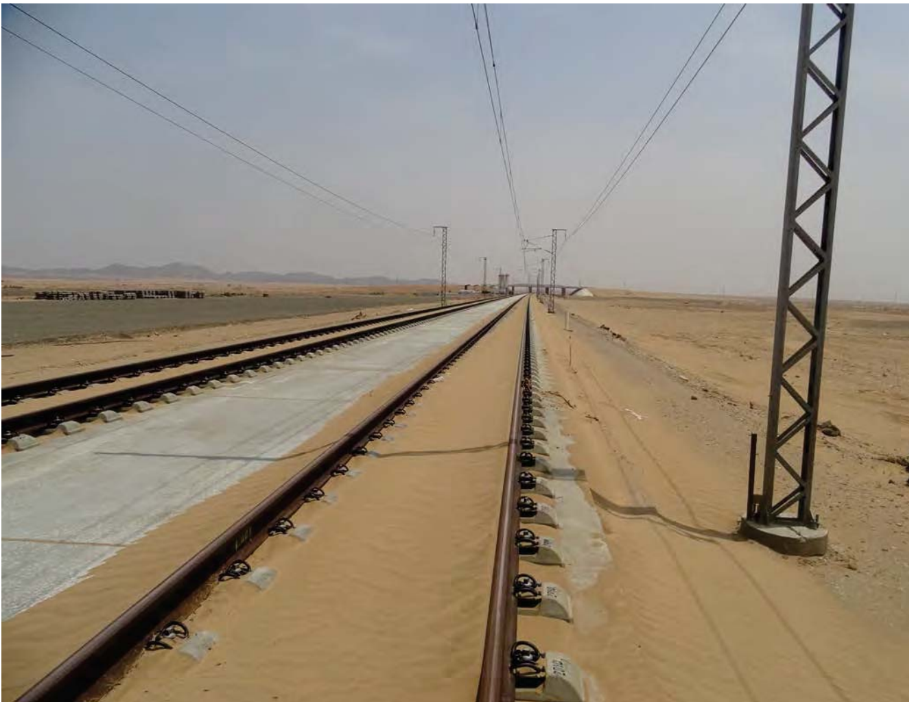
Railway Before sand cleaning (Desert Sand Trap on installation time)
